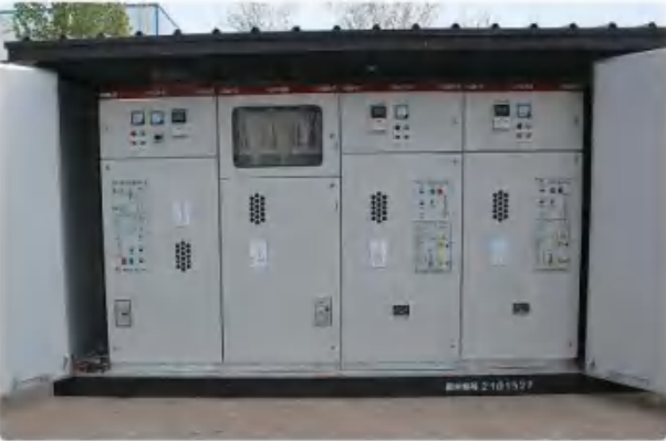
HXGN-12 环网开关柜 HXGN-12 ring network switch cabinet
